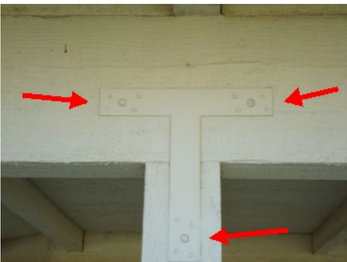
Each hole should have a lag bolt
